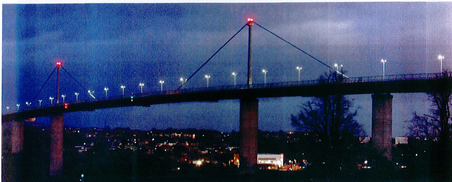
The completed Erskine Bridge: the new lighting scheme has extended luminaire and lantern design life, reduced maintenance costs and increased lighting levels
